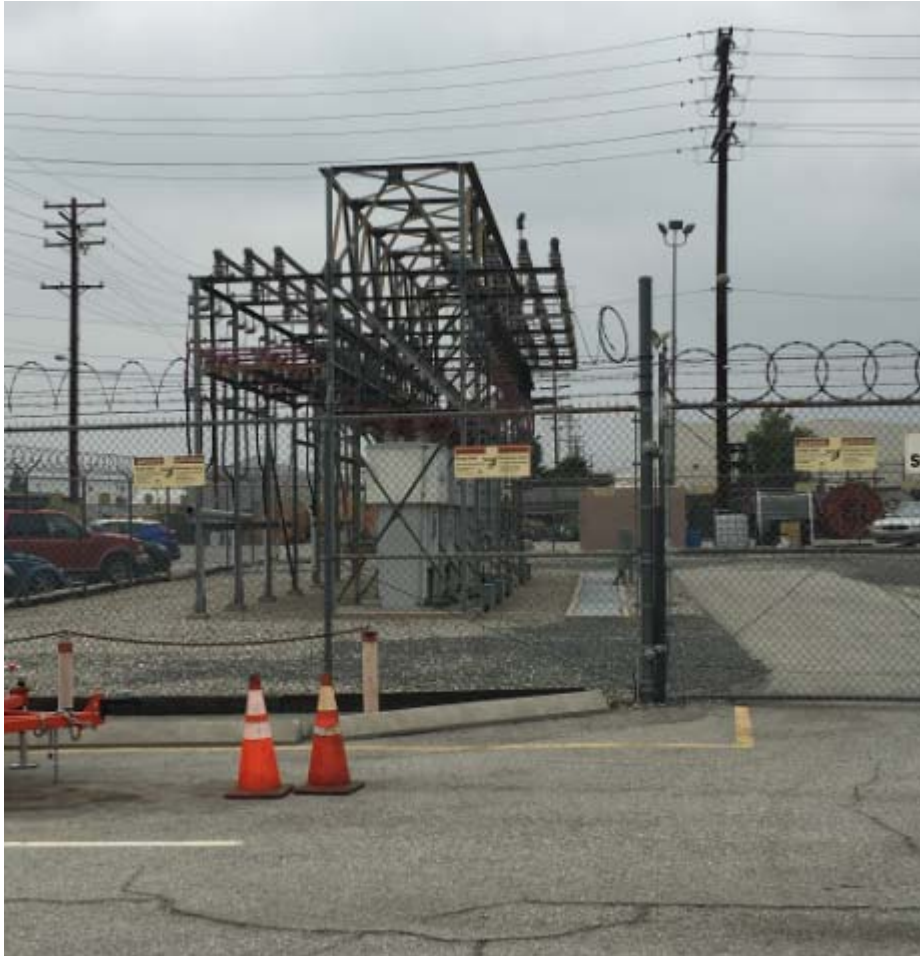
Picture 1: Existing adjacent switchrack, looking west
