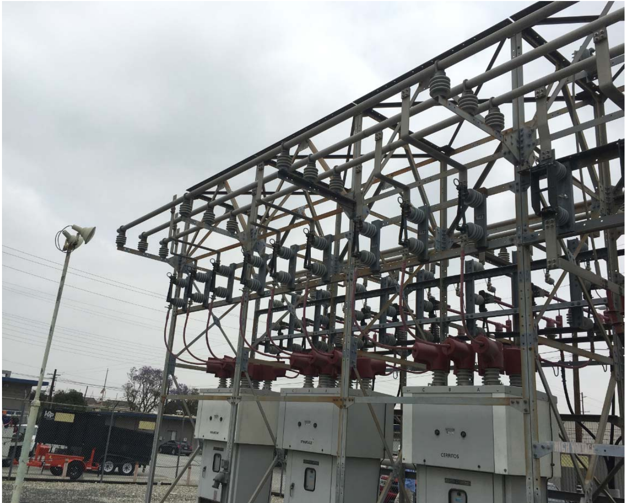
Picture 2: Existing adjacent switchrack, looking southeast
